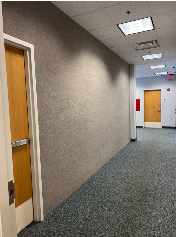
Main Area - CMU covered with felt
